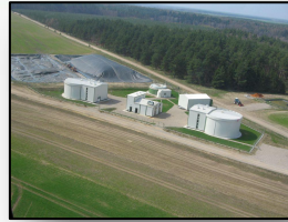
Biogas Plants (Cogeneration)
